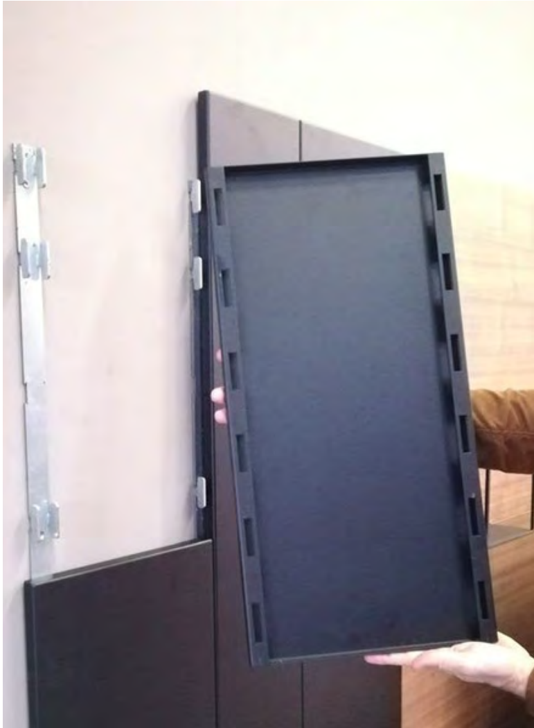
PANEL HAS SLOTS ON BACK FOR EASY AND FAST INSTALLATION
